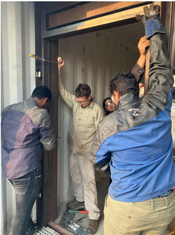
Figure 3: Installing entry unit. Neonomads, United Arab Emirates. Source: (Author 2023)
