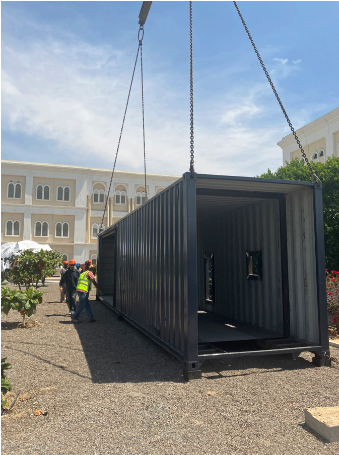
Figure 6: Craning container onto site. Neonomads, United Arab Emirates. Source: (Author 2023)
