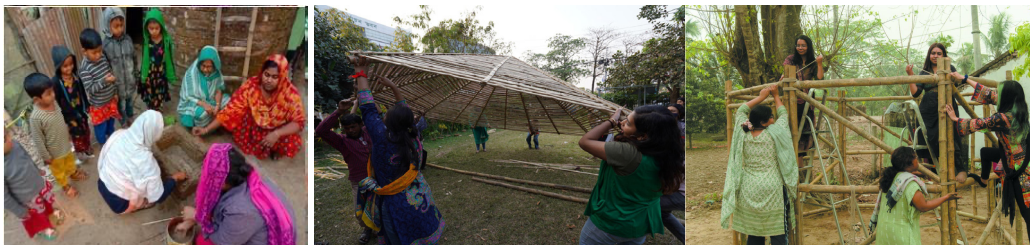
Figure 10: Women in the construction of zero carbon bamboo building. Source: (Author 2023)
