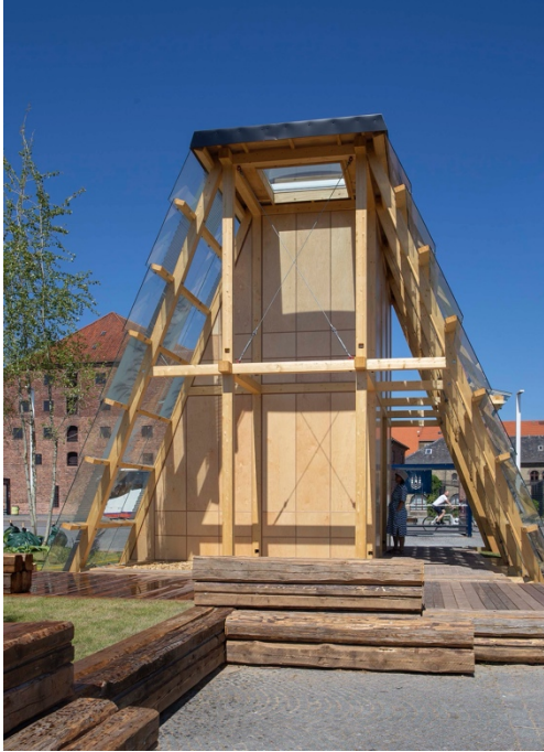
Picture 1: The 'Planetary Pavilion' by architectural office 'Lokal' exemplifies the integration of non-scalable elements within a scalable framework. Through participatory programming facilitated by a modular wood beam structure, the dwelling adapts to evolving user needs, fostering flexibility and inclusivity. Source: (Sandra Gonon 2023)
