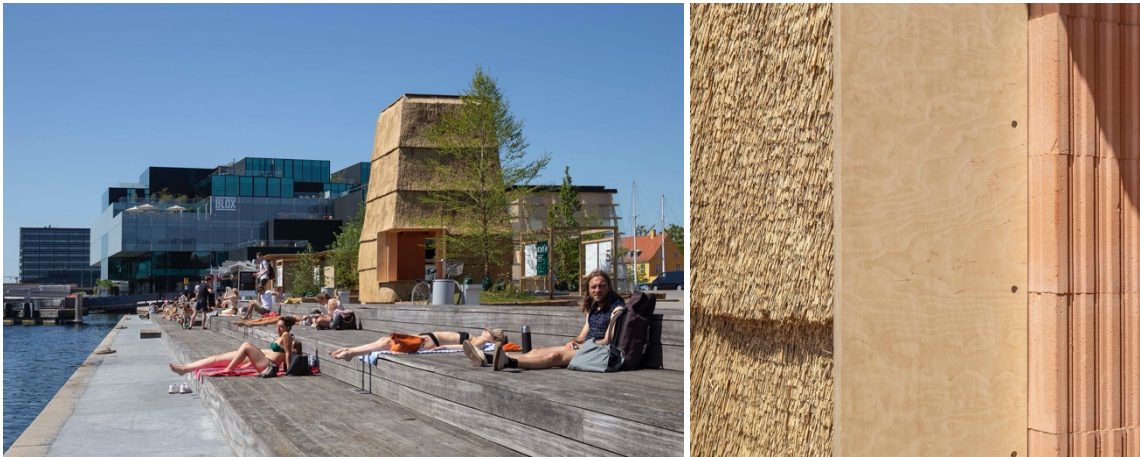
Picture 4 and 5: The thatched facade of the pavilion 'Thatched Bricks' by the offices 'Leth & Gori' and 'Rønnow' in collaboration with 'CINARK'. Thatching is a craft that today is done by a skilled craftsman utilizing a variety of 'transparent technologies', such as the thatcher's 'leggett'; a flat board attached to a handle used to drive the reeds into place. In this instance, the façade was constructed off-site as façade-elements, and subsequently transported for on-site montage. This allowed for a somewhat 'scalable' production, enabling a broader variety of reed quality to be used, as well as providing logistical potentials in terms of improved workflow and sheltering. In combination with the sophisticated insulating bricks, it demonstrates the possibility of working within the spectrum of 'transparent' and 'opaque' technologies. Source: (Sandra Gonon 2023)
