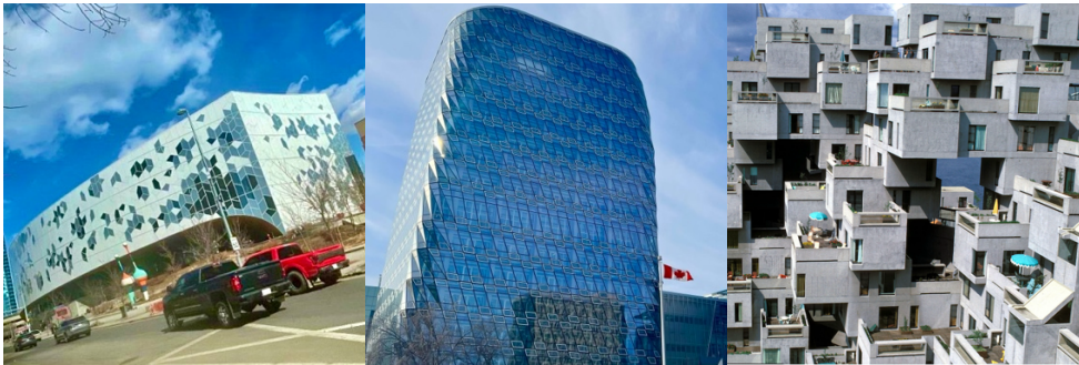
Figure 1: Selected contemporary architectural case studies. From left to the right: the new Calgary Central Library (Architects: Snohetta + DIALOG, Location: Calgary, Alberta, Canada), The MacKimmie Tower (Architects: Ron Thom, renovated by DIALOG, Location: Calgary, Alberta, Canada), and Habitat 67 (architect: Moshe Safdie, Location: Montreal, Quebec, Canada). Source (From left to right): (Sinclair 2023) (Bahonar 2024) (Gabrieled 2013)
