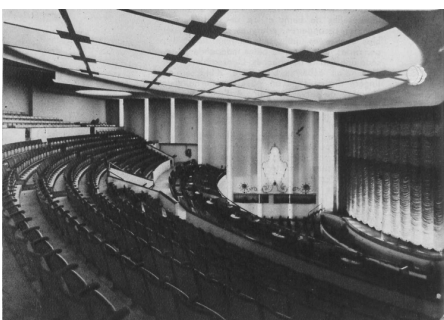
Figure 1: Magazine article photograph showing the original chequerboard rooflight. Source: (BATIR 61, December 1937)
