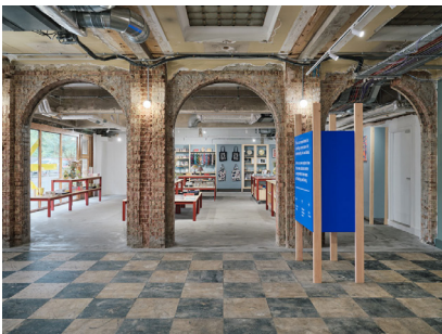
Figure 4: Stripped back interior with exposed brickwork, Charleston in Lewes. Source: (Material Cultures / Henry Woide 2023)
