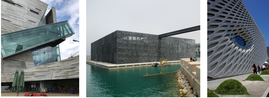
Figure 1: Selected precast projects. From left to right, Perot Museum of Nature and Science, with traditional architectural precast concrete; Museum of Civilizations of Europe and the Mediterranean (MuCEM), with ultra-high performance concrete (UHPC); The Broad, with glass-fiber reinforced concrete. Sources (from left to right): (Cutrer 2017, Harald 2013, Author 2016)
