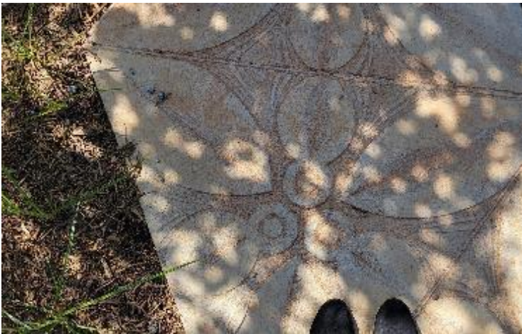
Figure 6: The team designed and fabricated custom concrete stamps informed by patterns printed on fabric at the Bleachery. These were used to stamp patterns along the pathway of the plaza. Source: (Dickey 2023)
