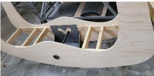
Figure 8: Prototype of rocker and anchor box for testing the prevention of overturning while allowing for rocking motion. Source: (Dickey 2023)
